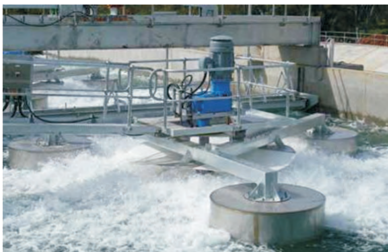
Fig 18.6 Aeration of clarified water
